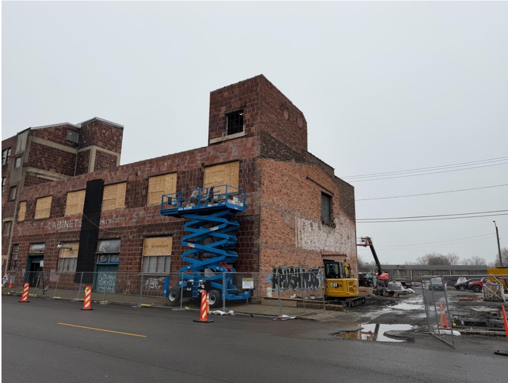
S-3: Primary (North) Façade and West Elevation of 619 Exchange, facing SE
