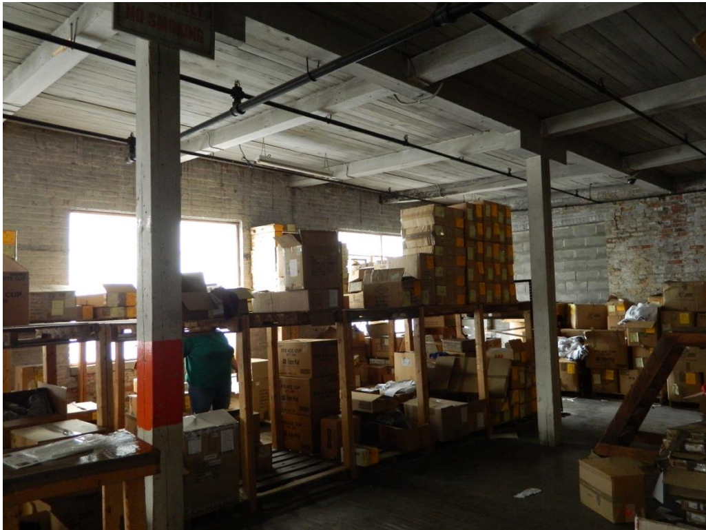
D-8: 4 th Floor 629-659 Exchange, facing SE
