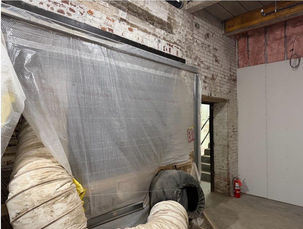
B-13: 2 nd Floor 629-659 Exchange, facing NW
