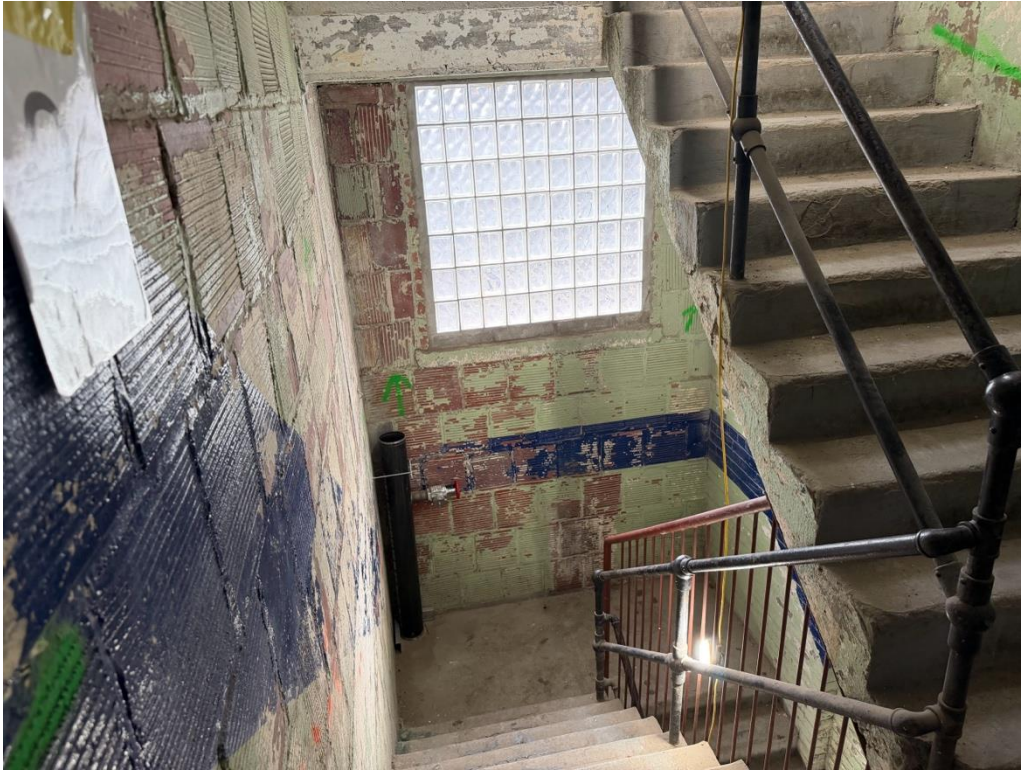
B-11: 2 nd Floor 619 Exchange, facing N
