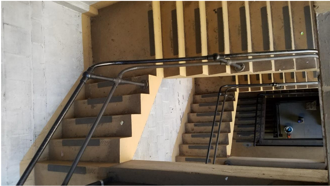
D-7: 4 th Floor 629-659 Exchange, facing S
