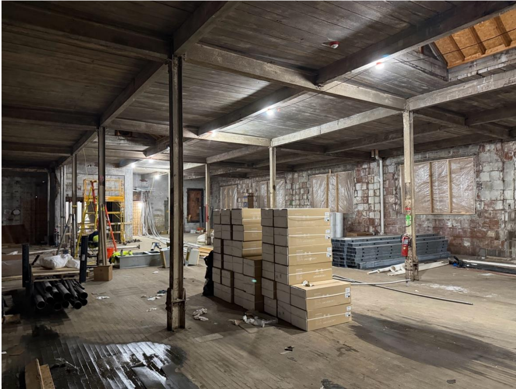
B-7: 2 nd Floor 619 Exchange, facing SE
