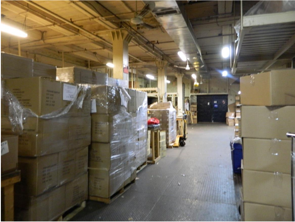
A-11: 1 st Floor 629-659 Exchange, facing W
