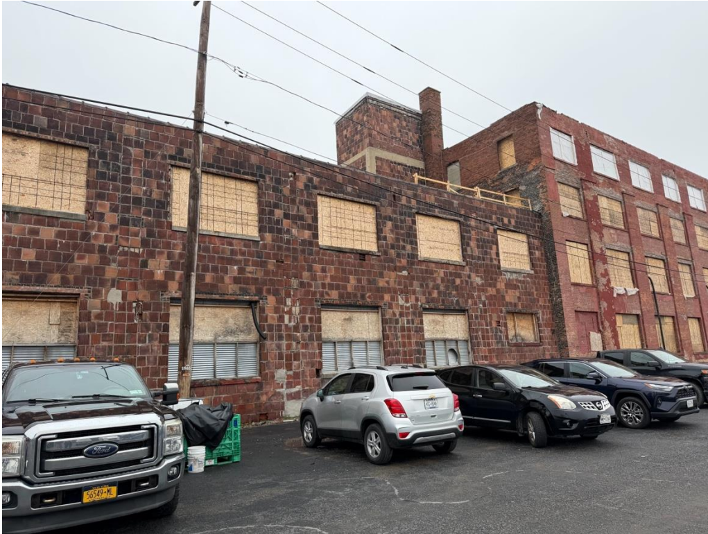
S-7: South Elevation of 619 Exchange, facing NE
