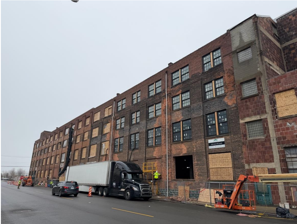
S-11: Primary (North) Façade of 629-659 Exchange, facing SE
