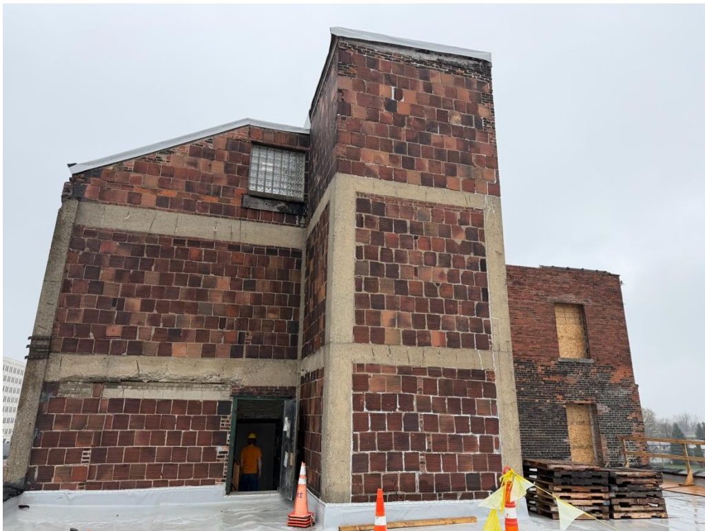
S-12: Roof of 619 Exchange, showing stair tower and portion of 629-659 Exchange brick wall, facing SE
