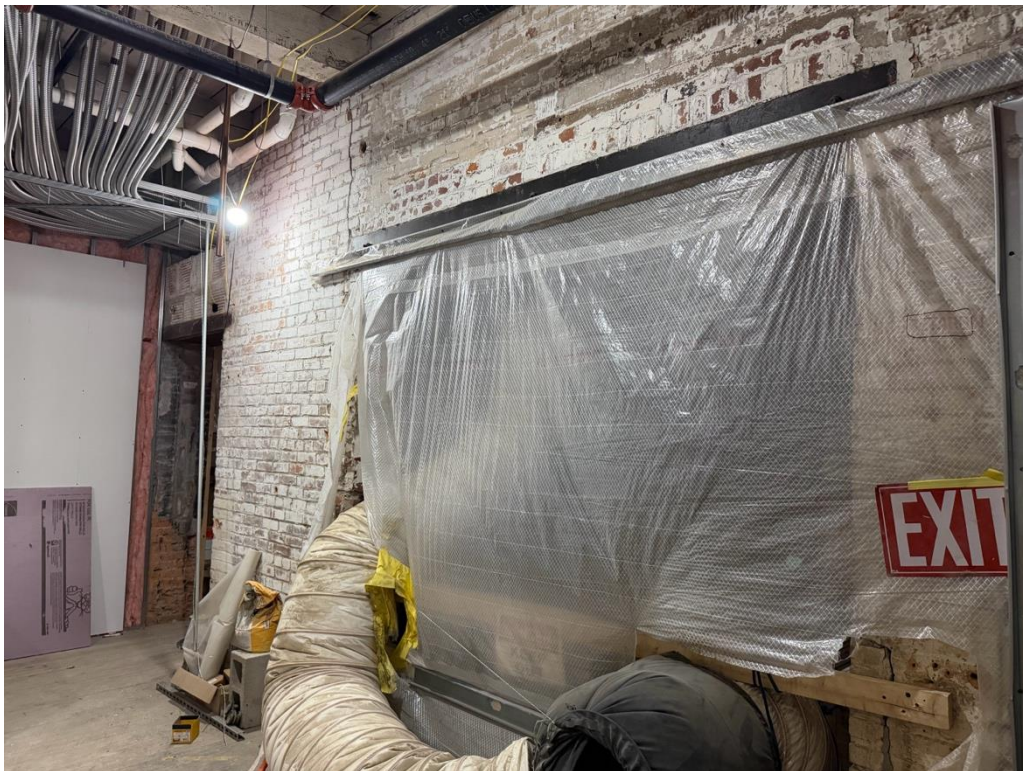
B-12: 2 nd Floor 629-659 Exchange, facing SW
