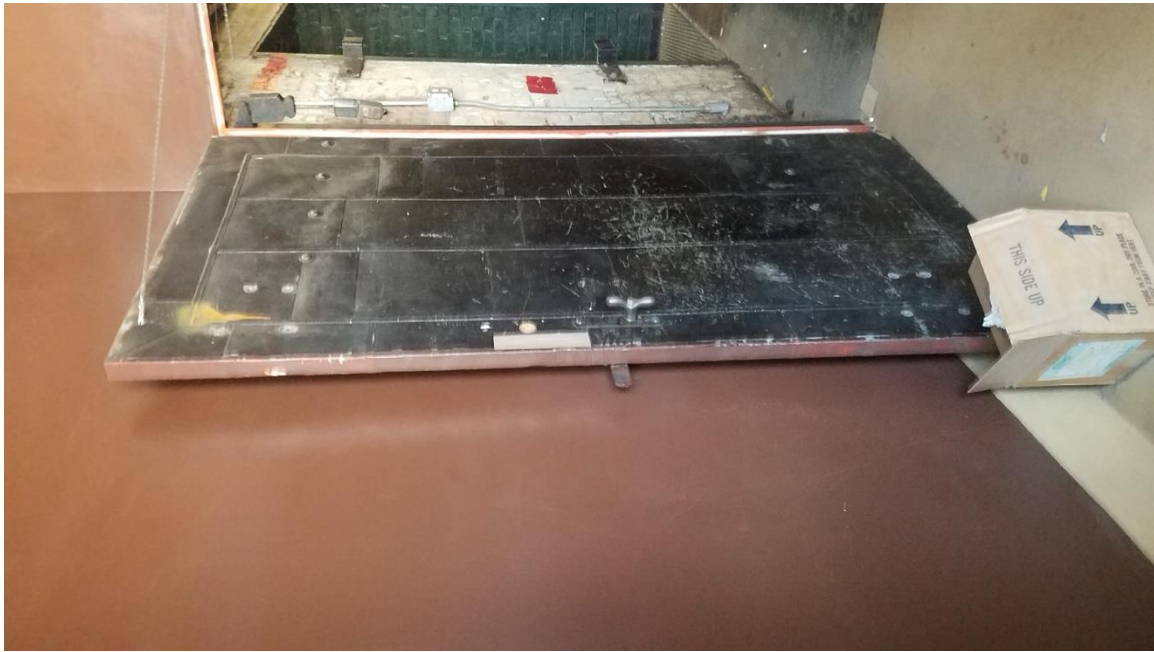
B-19: 2 nd Floor 629-659 Exchange, facing SE
