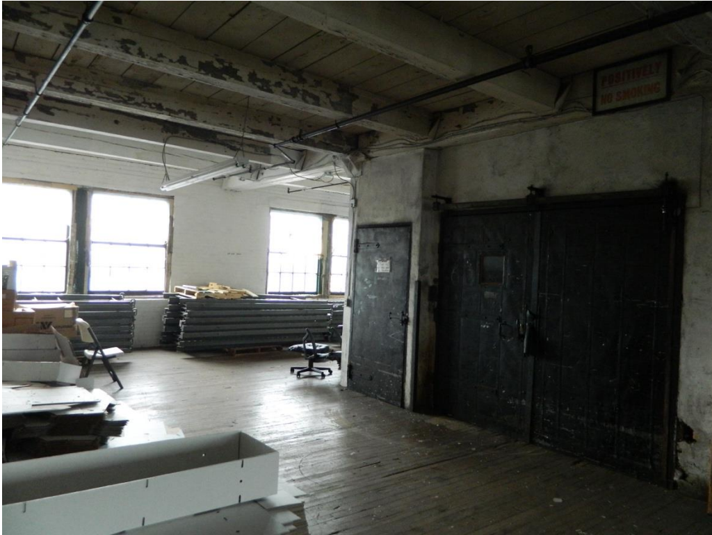
C-7: 3 rd Floor 629-659 Exchange, facing SW
