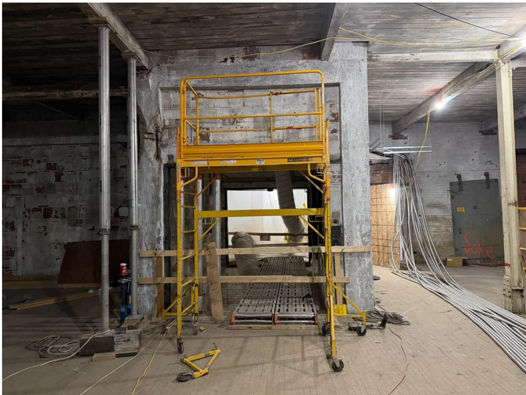
B-4: 2 nd Floor 619 Exchange, facing E
