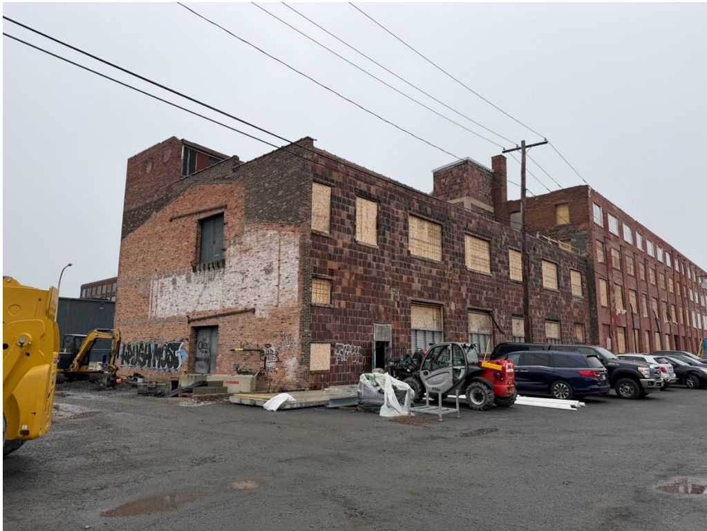
S-6: South and West Elevations of 619 Exchange, facing NE
