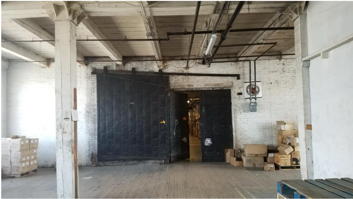
B-15: 2 nd Floor 629-659 Exchange, facing E
