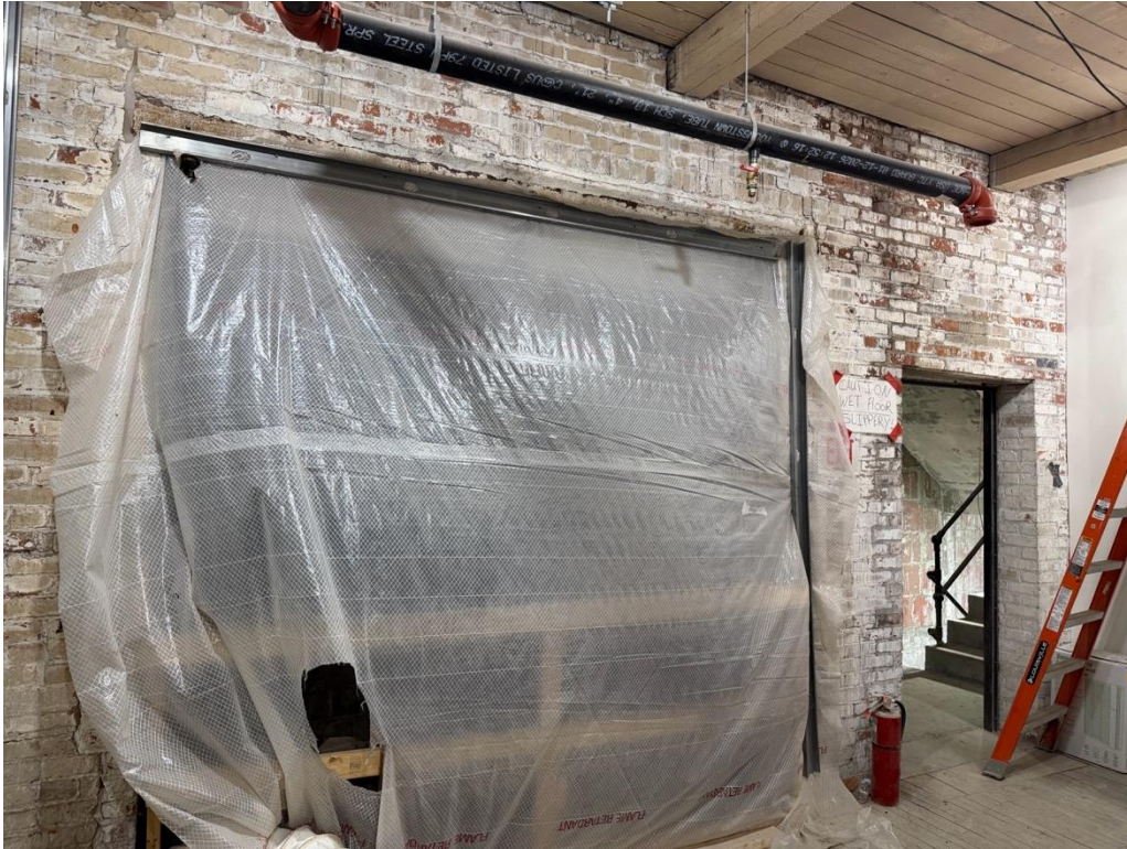
D-1: 4 th Floor 629-659 Exchange, facing NW
