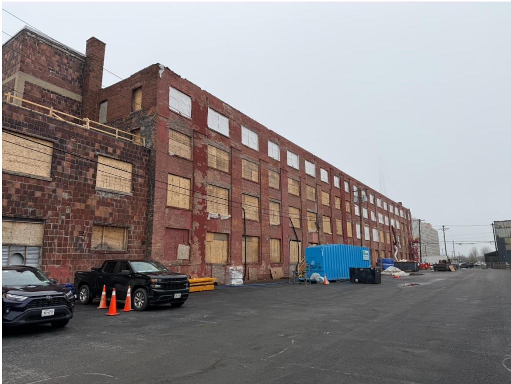
S-8: South Elevation of 629-659 Exchange, facing NE
