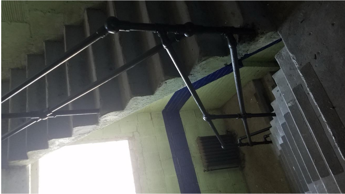
C-3: 3 rd Floor 629-659 Exchange, facing NW
