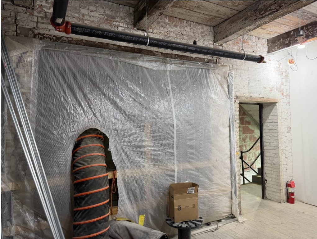
C-1: 3 rd Floor 629-659 Exchange, facing NW
