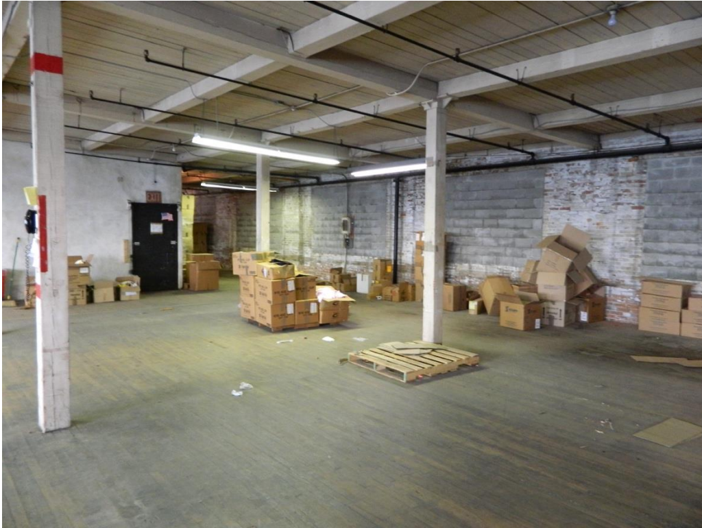
D-3: 4 th Floor 629-659 Exchange, facing SE
