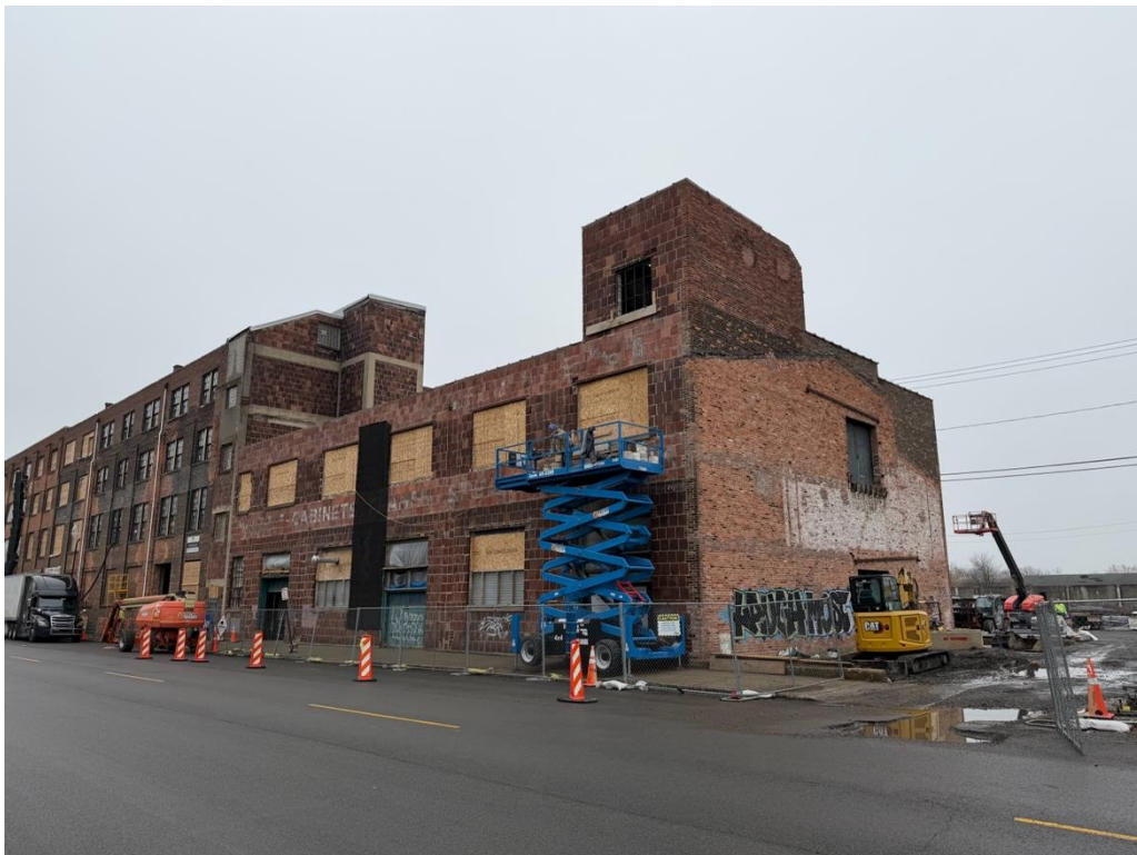
S-4: Primary (North) Façade and West Elevation of 619 Exchange, facing SE
