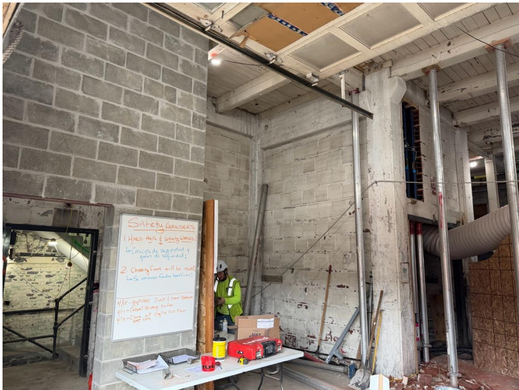
A-2: 1 st Floor 619 Exchange, facing SE
