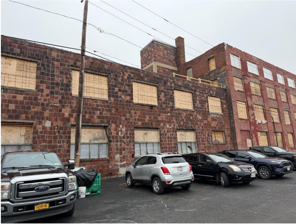
S-7: South Elevation of 619 Exchange, facing NE
