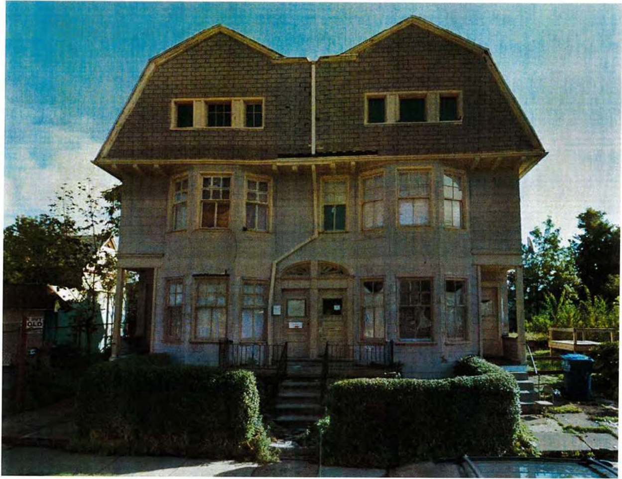
Photo of the building in 2011, depicting the façade without the vinyl clapboard between windows on the third story. While the current paint configuration deemphasizes historic detailing, the historic appearance is more evident with neutral colors.
