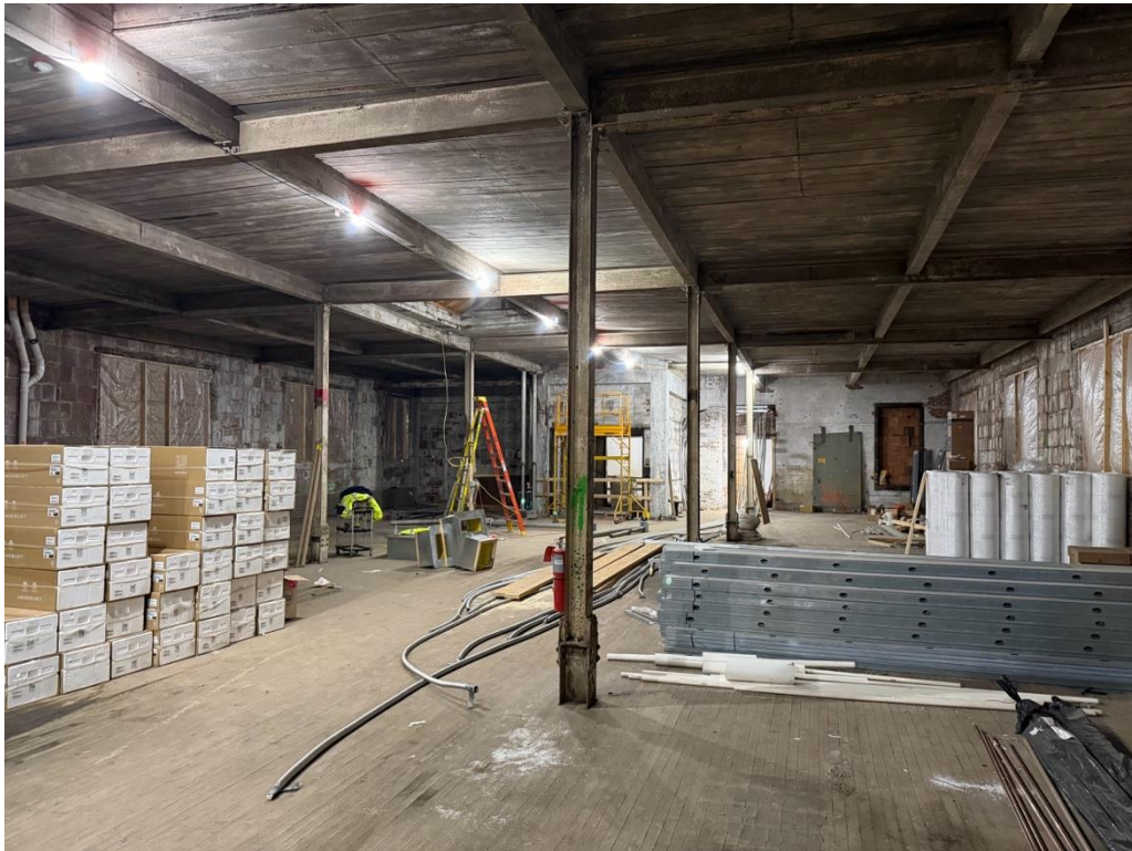
B-10: 2 nd Floor 619 Exchange, facing NE
