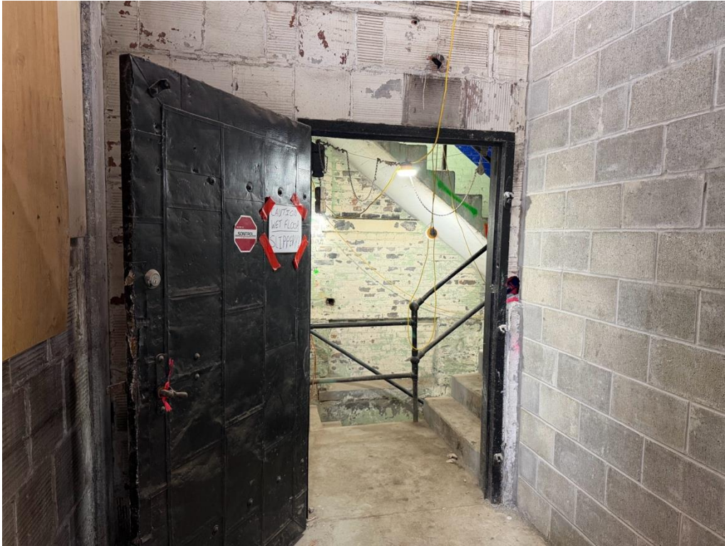
A-3: 1 st Floor 619 Exchange, facing E
