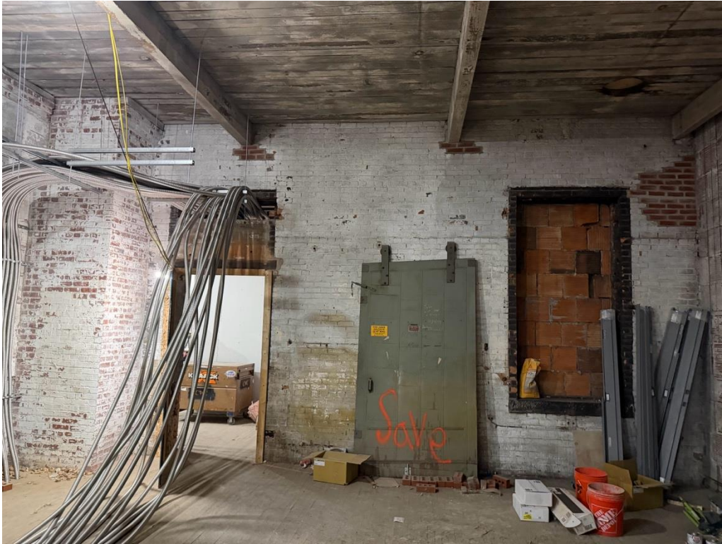
B-3: 2 nd Floor 619 Exchange, facing E
