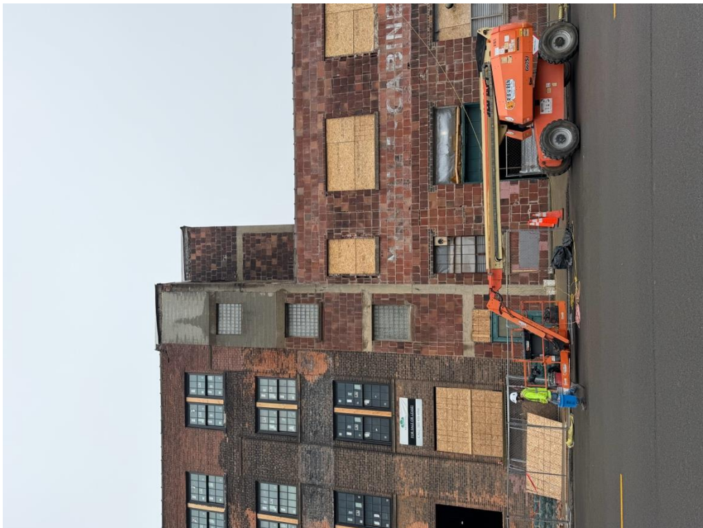
S-2: Primary (North) Façade of 619 Exchange, showing where abuts 629-659, facing S
