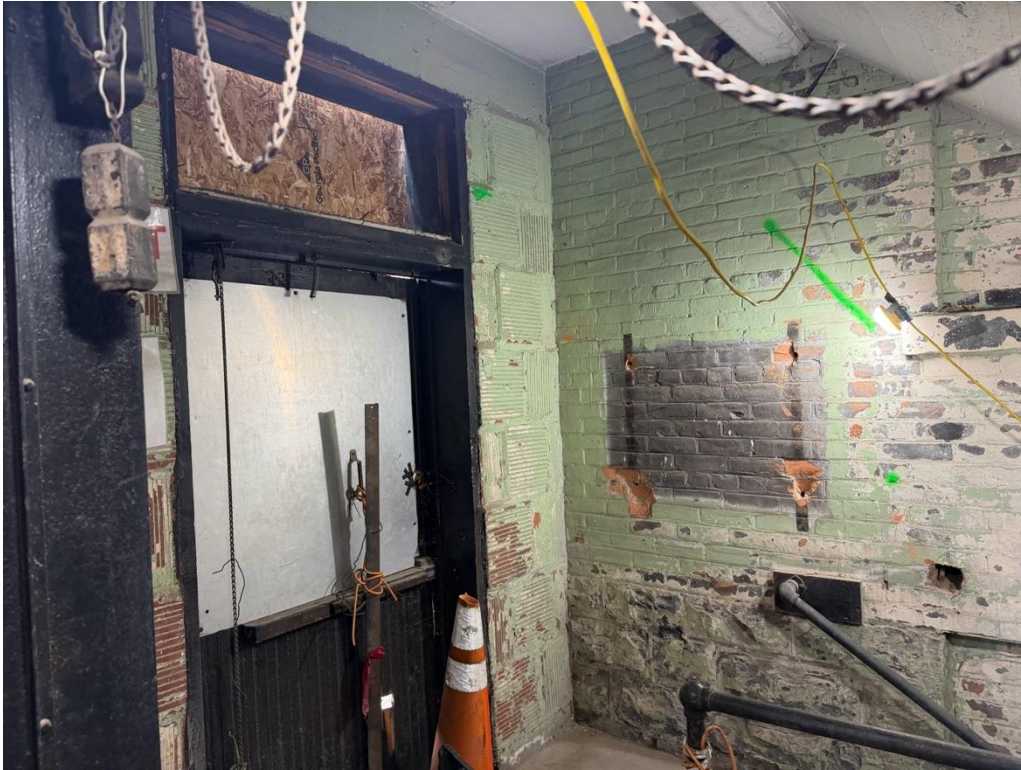
A-1: 1 st Floor 619 Exchange, facing NE
