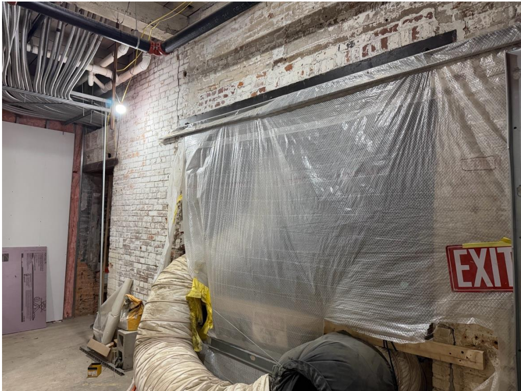
B-12: 2 nd Floor 629-659 Exchange, facing SW
