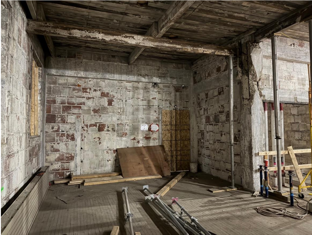
B-5: 2 nd Floor 619 Exchange, facing E
