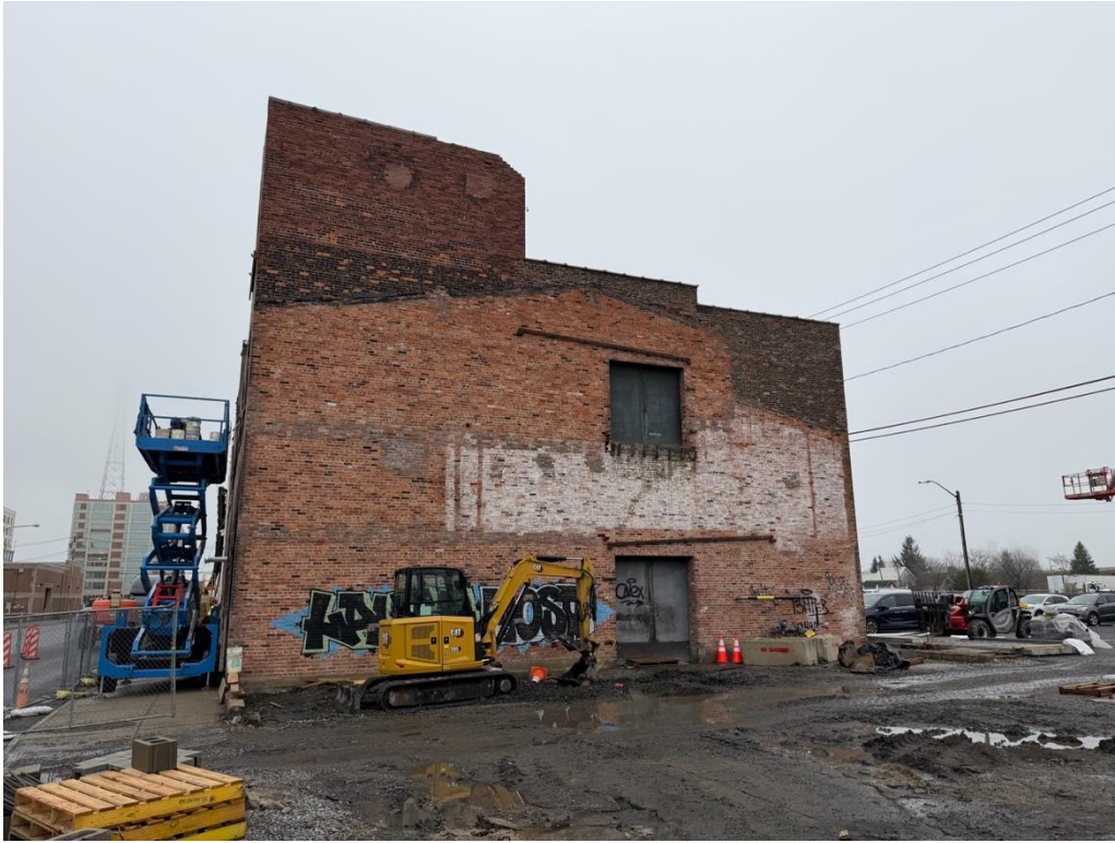
S-5: West Elevation of 619 Exchange, facing E
