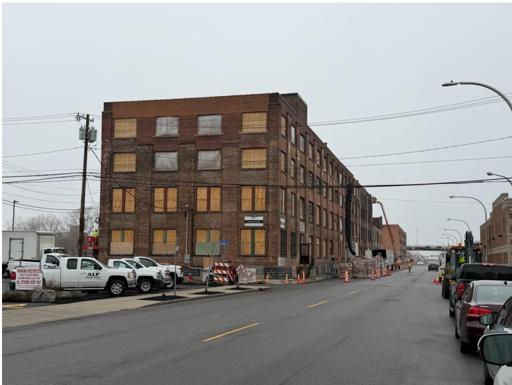
S-10: Primary (North) Façade and East Elevation, facing SW
