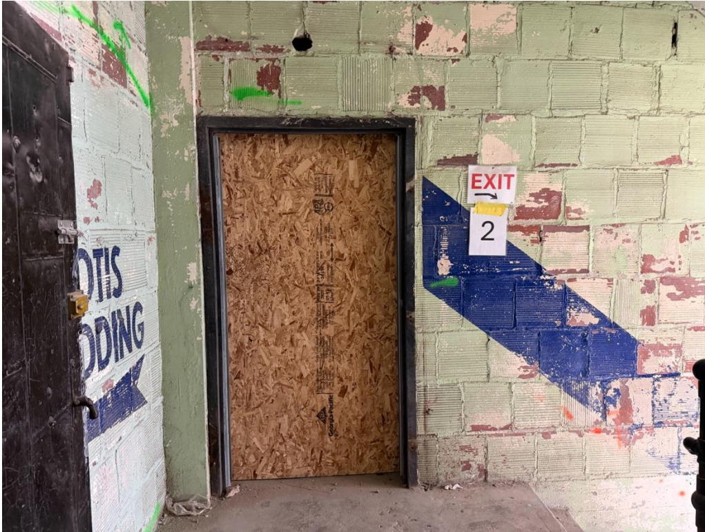
B-1: 2 nd Floor 619 Exchange, facing W
