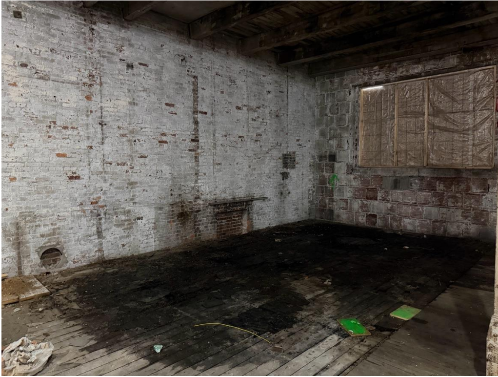
B-9: 2 nd Floor 619 Exchange, facing NW
