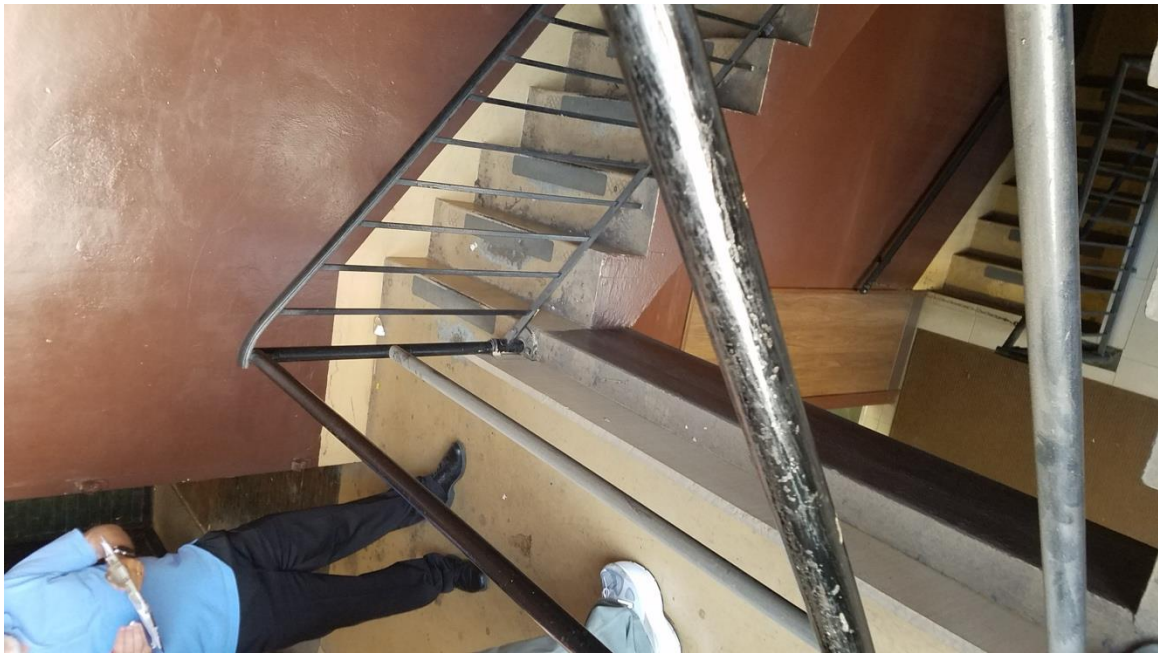
B-18: 2 nd Floor 629-659 Exchange, facing S
