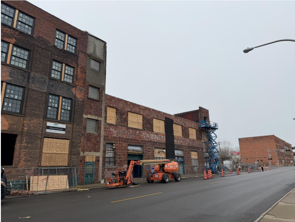
S-1: Primary (North) Façade of 619 Exchange, facing SW
