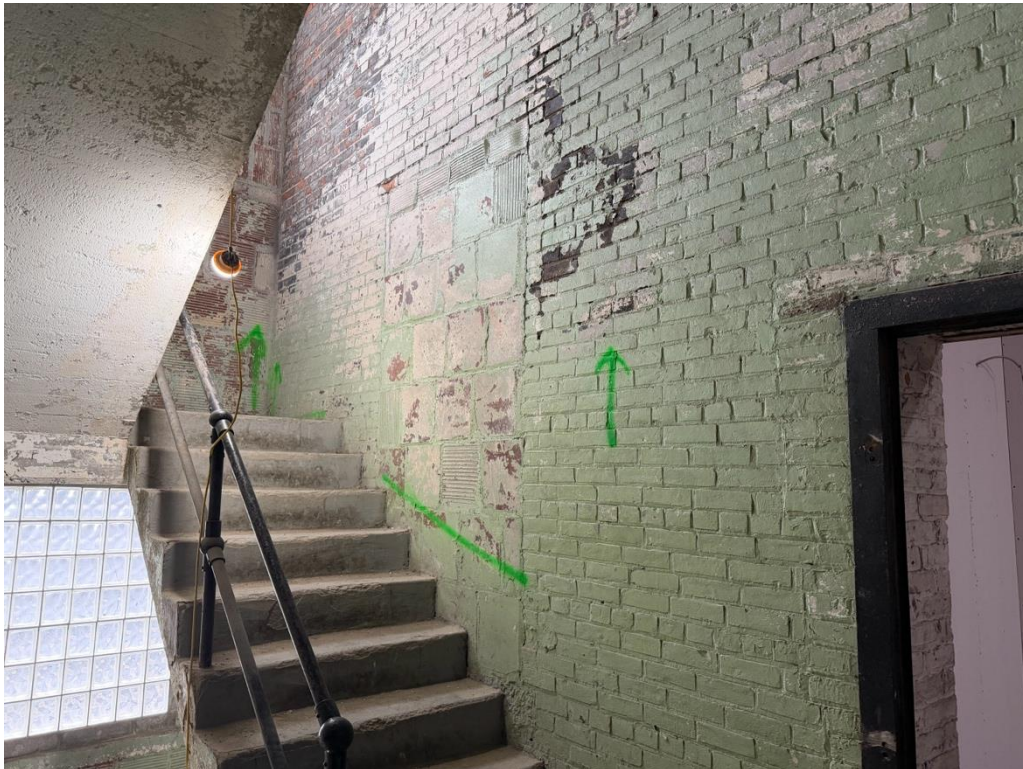
B-2: 2 nd Floor 619 Exchange, facing NE
