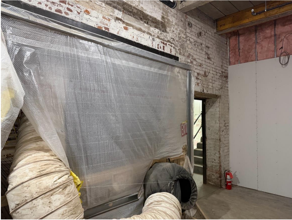
B-13: 2 nd Floor 629-659 Exchange, facing NW
