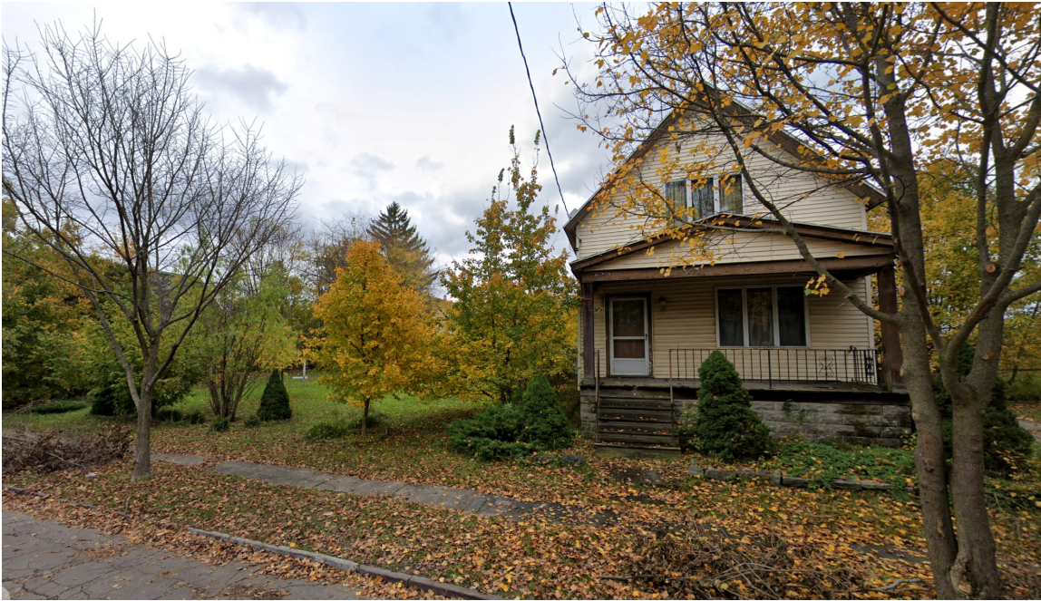
Photo 1: View from the street (Armbruster St) looking at 11 Armbruster Street.
