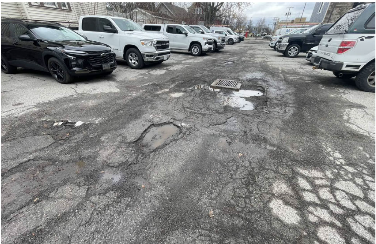
Parking Lot Catch Basin/Drain
